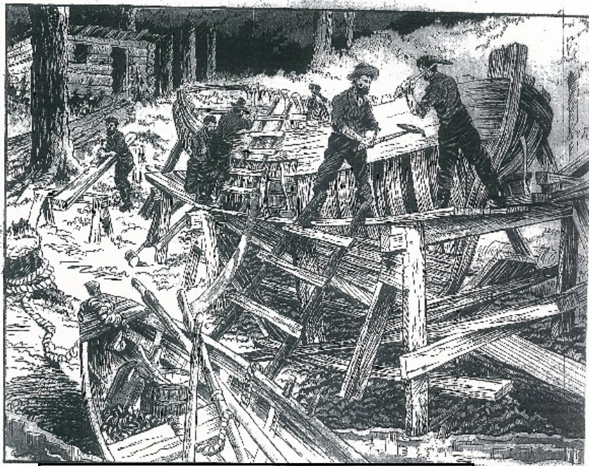
Above drawing of the ship being constructed is from the May 18, 1941 edition of The Oregonian
